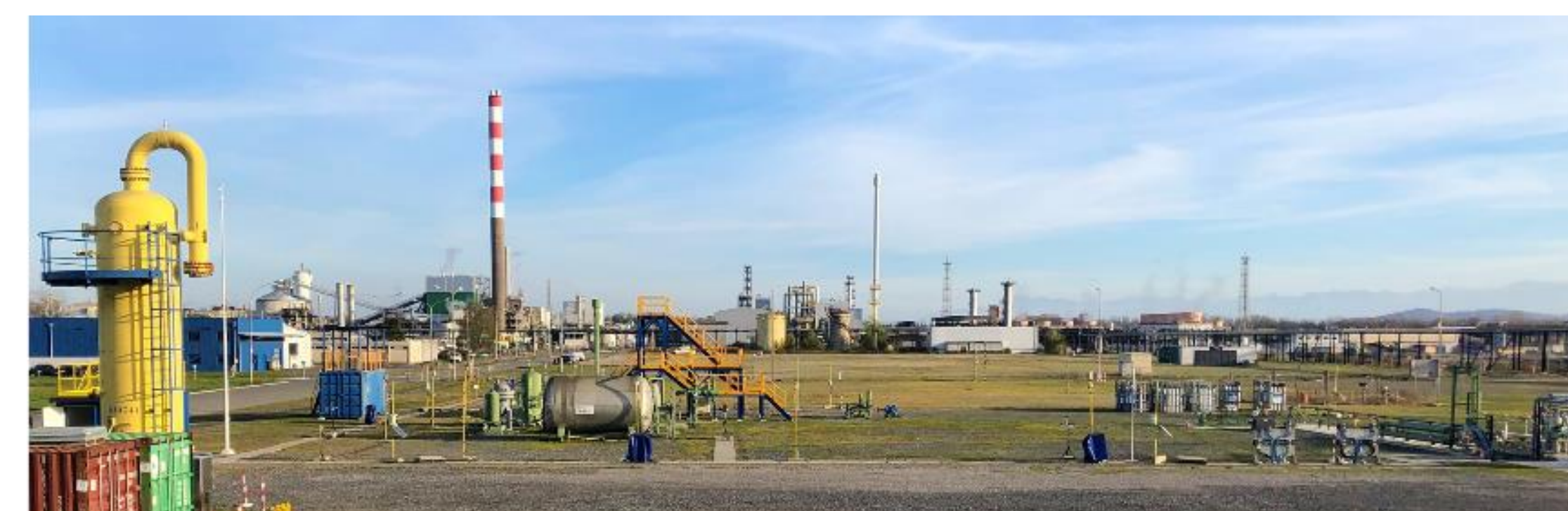
Total Energies' TADI facility (foreground) with host industrial site in background.
