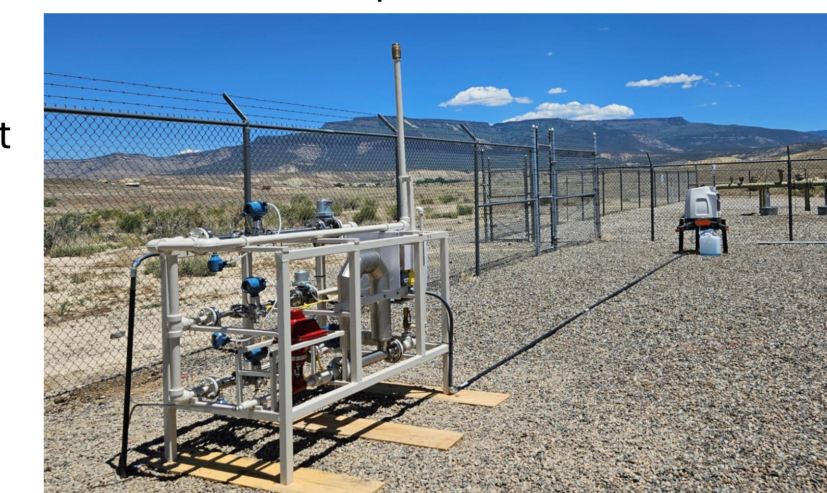
Figure 7: Satellite release rig set up at Kinder Morgan's testing location
