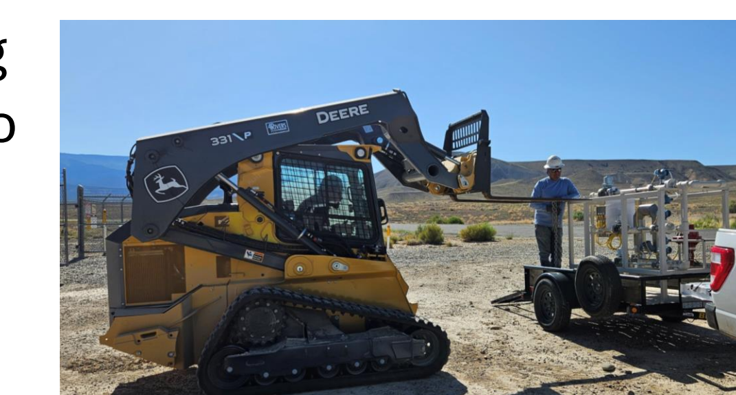
Figure 8: Installation of the release rig at the Kinder Morgan testing location
